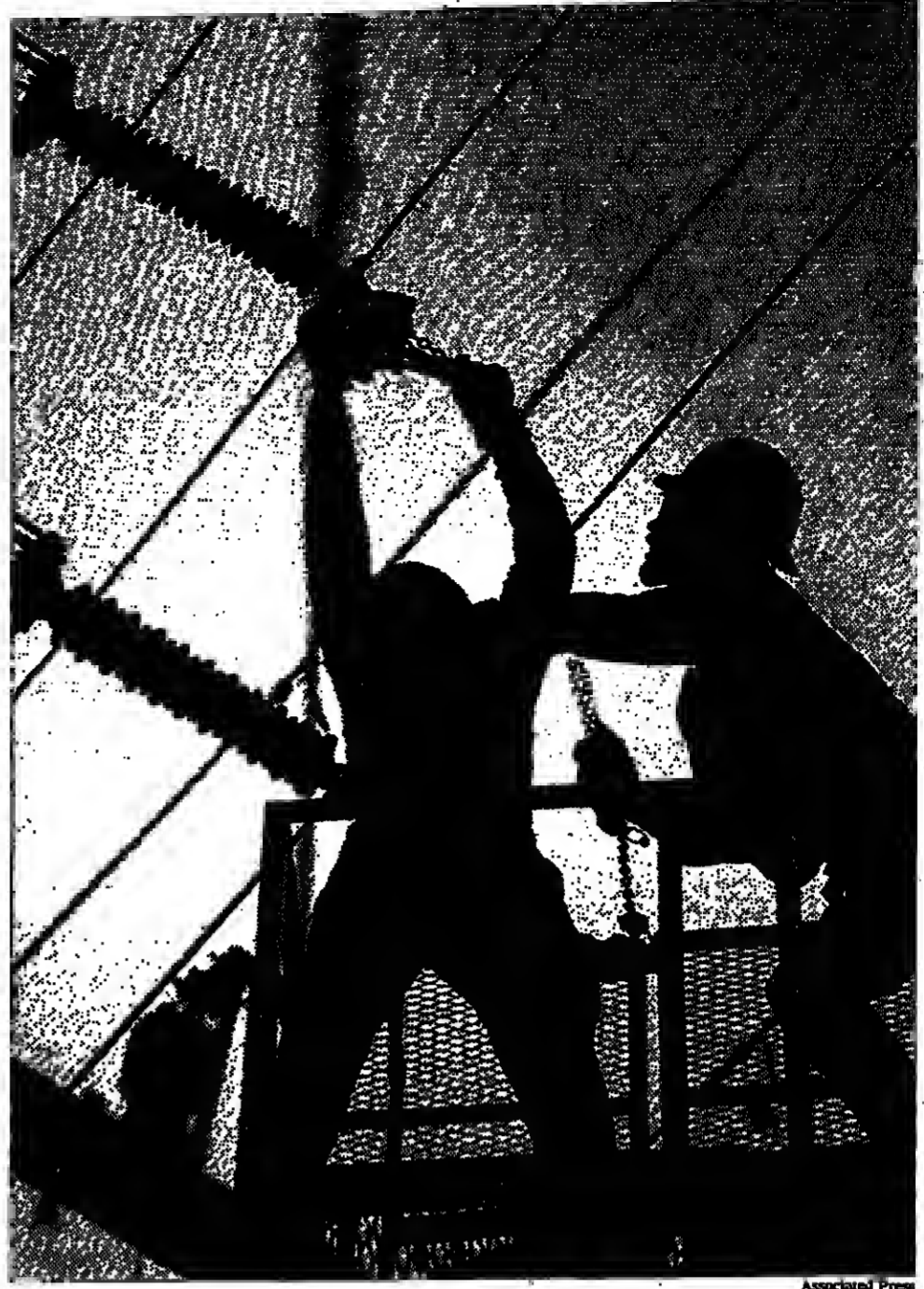
Workers repairing lines in California, a state set to deregulate electric monopolies.
